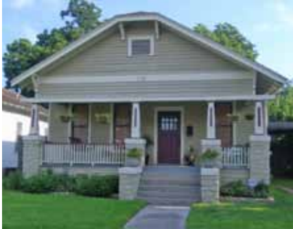
Design guidelines provide useful information about maintaining historic properties.
