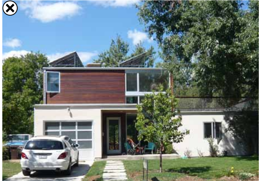
✗ This building is not compatible with the Houston Heights historic districts context.
