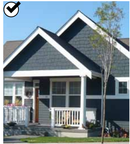
Construct a new building to be compatible with contributing buildings in the context area.
