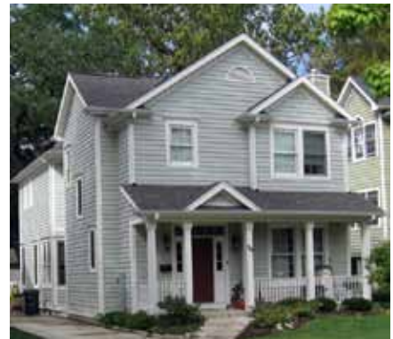
The mass & scale of this new infill building would be appropriate in some Houston Heights contexts. However, the foundation is inappropriate.
