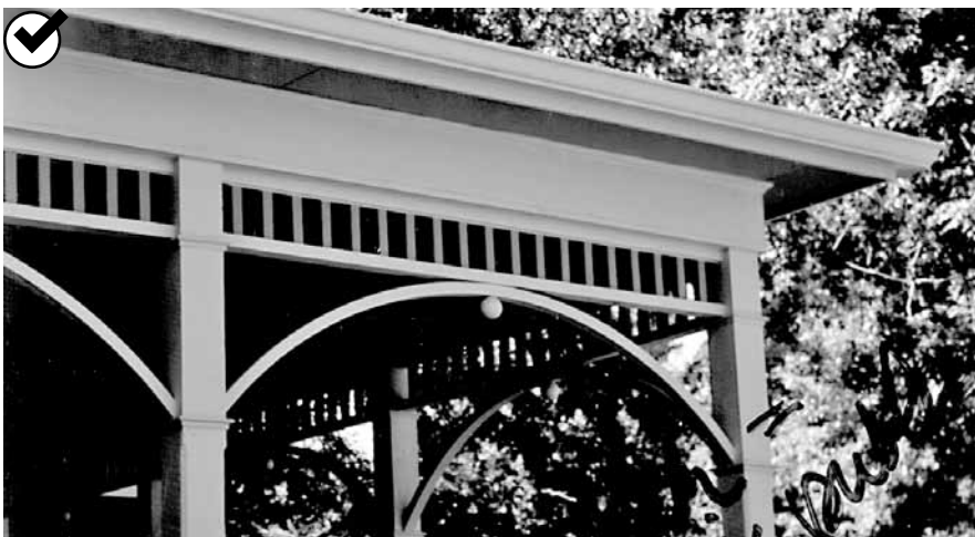
Use new interpretations of porch columns, balustrades, rafter ends, and details to distinguish new from old.
