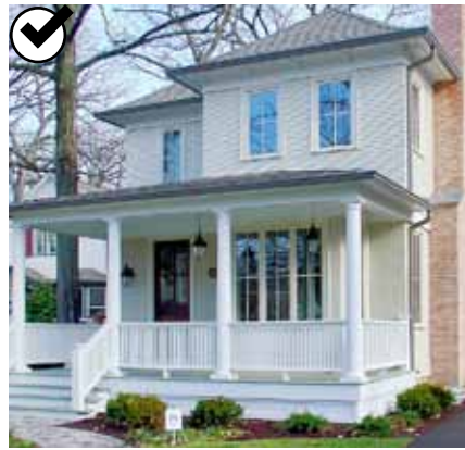
A hip roof, simple building form and raised porch are appropriate features on this building. Porch and eave height are scaled appropriately.
