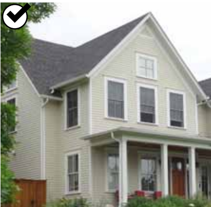
✓ Use materials that are similar in dimensions, profile, and finish to traditional materials.
