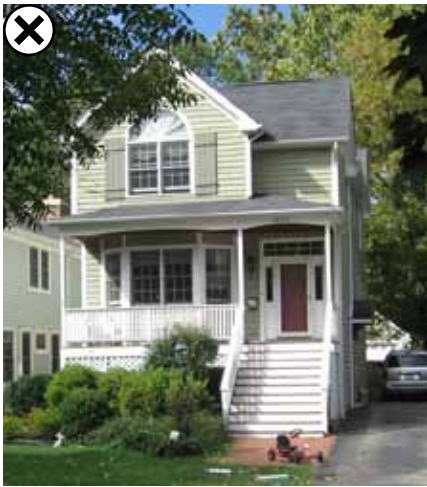
The raised foundation, shutters and windows on this new infill building are inappropriate. The foundation is too high, the windows are too elaborate and shutters are fake.
