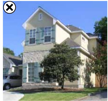
This new infill building would be incompatible within the Houston Heights Districts. The windows and building massing is out of proportion. Stone is also incompatible within the districts.
