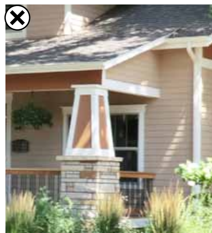
This column is out of scale with the porch.
