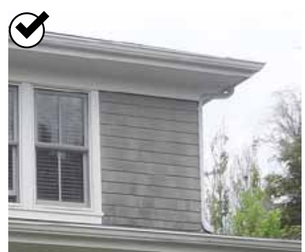
Use an eave overhang that appear similar to those seen on historic buildings in the context area.
